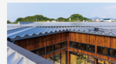
Solar power generation equipment at MUJI Karatsu
